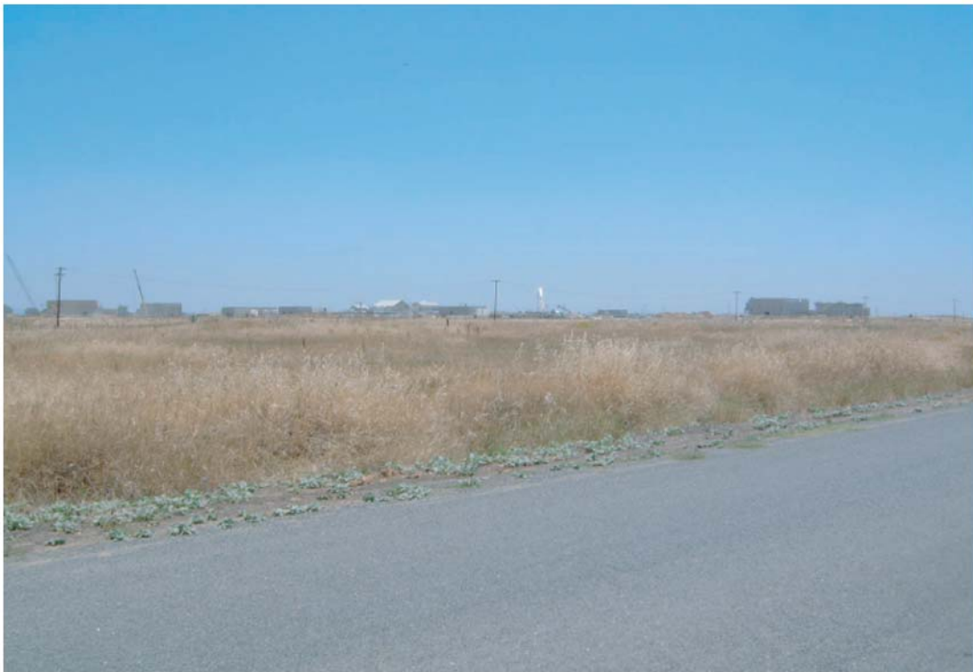
F. Wastewater Treatment Plant
